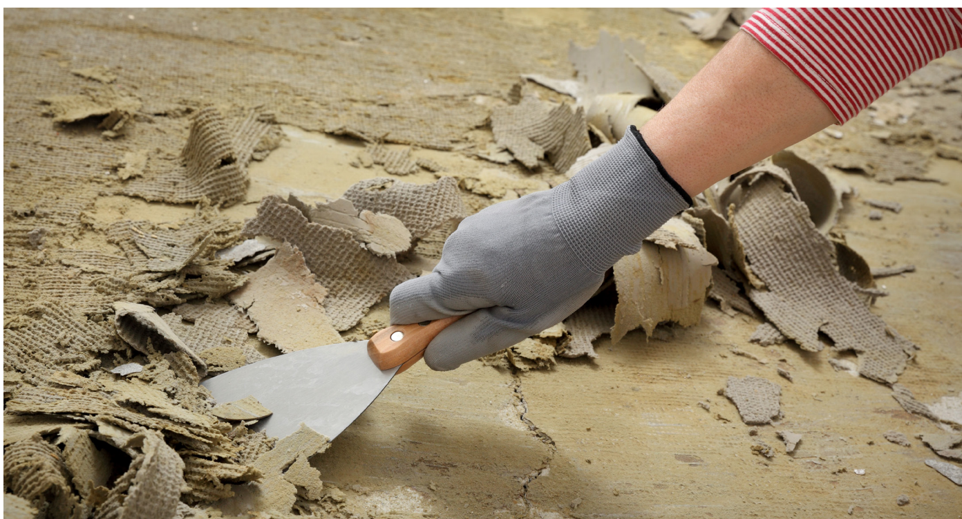
Photo: With the right PSA, no extra cleaning work is required when removing the flooring
